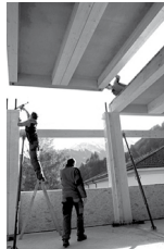
Installation of prefabricated concrete deck and timber beam floor panels
