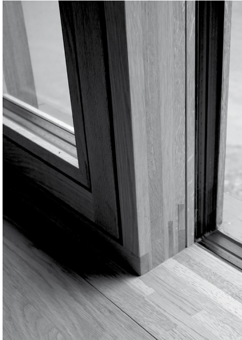
Detail view of oak framed window unit
